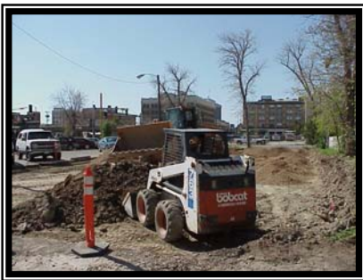
The new parking lot, a work in progress.
